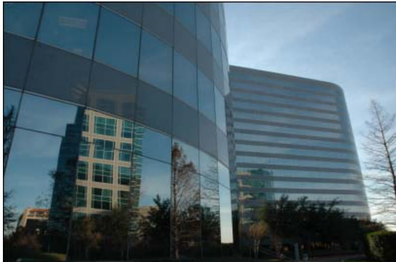
A typical Office Property in the Area.
